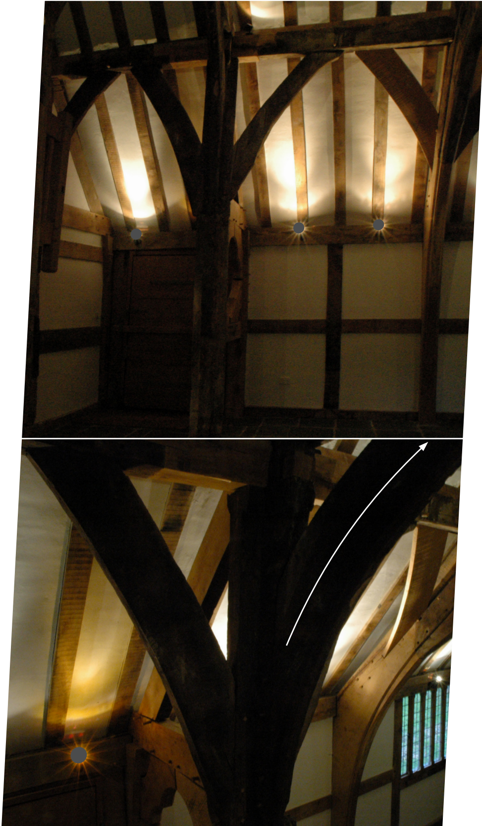
Appendix 9 Interior Original and modern timbers Spere post, left, and cruck, right, bracing to arcade plate Spere post, left, arcade bracing and hall arch (arrowed)
