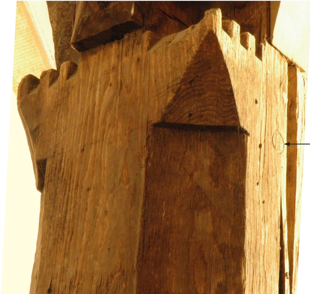
Appendix 10 Interior Original timbers Cusped cruck head Spere post crenelated capital Compass race knife circle carpenter's assembly mark
