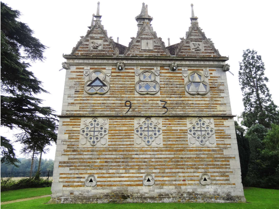
Triangular Lodge north facade
